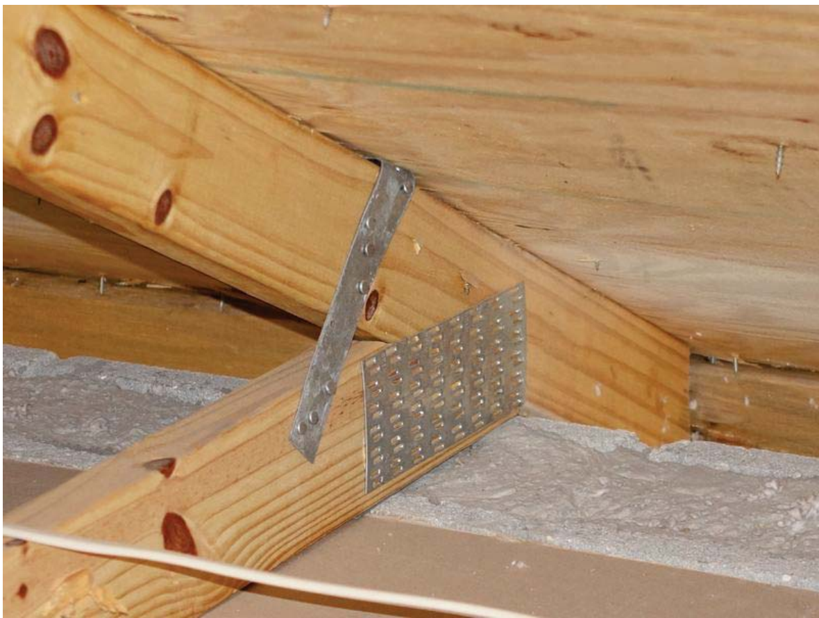
ROOF TO WALL - STRAPS BACK SIDE - OK
