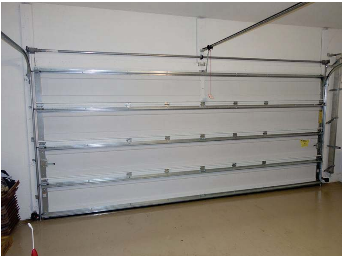
HURRICANE BRACED GARAGE DOOR OK
