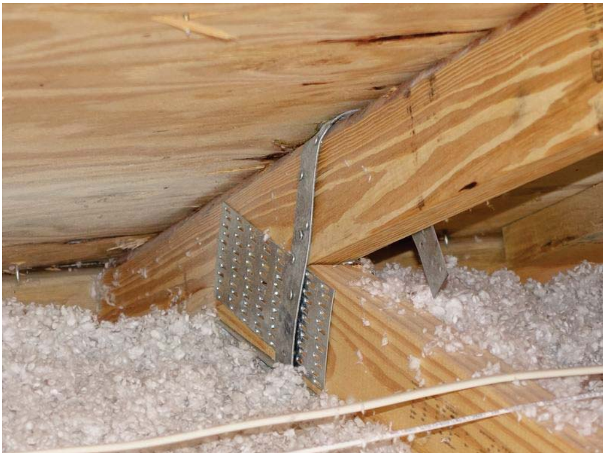
ROOF TO WALL - STRAPS FRONT SIDE - OK
